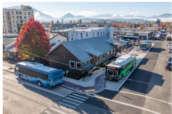
Figure 5-1 - JCT Transit Center in Downtown Grants Pass
