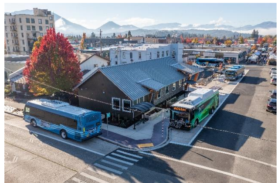
Figure 5-1 - JCT Transit Center in Downtown Grants Pass
