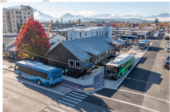
Figure 5-1 - JCT Transit Center in Downtown Grants Pass
