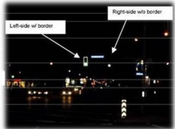
Exhibit 8 Example of signal head visibility with and without reflective backplates.
