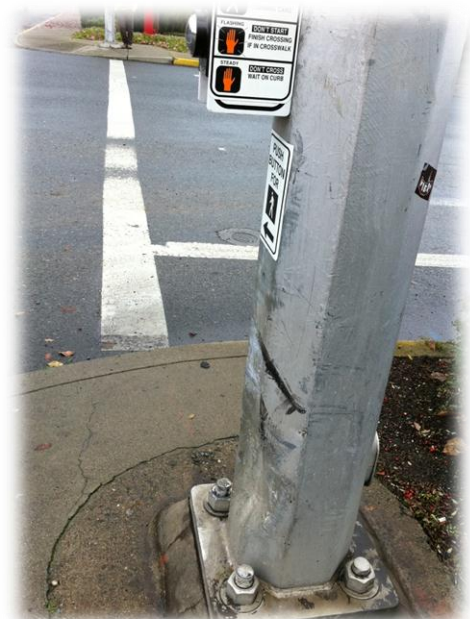
Exhibit 39 Signal poles damaged from vehicle hits
